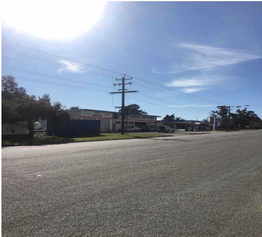
Image 1: Shipping Container on Road Reserve without Consent or Tie down on Entrance to Town. RU5 Village Zone
