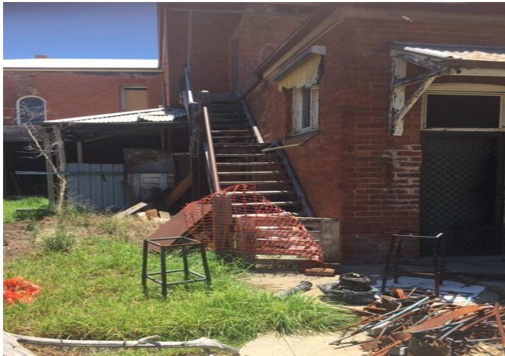
Image 1: Engineers Certified Rear Stair Barricading
