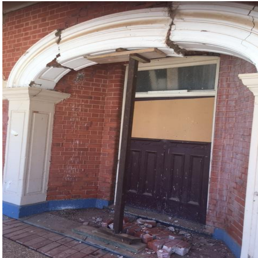
Image 2: Engineers Certified Support of Front Archway
