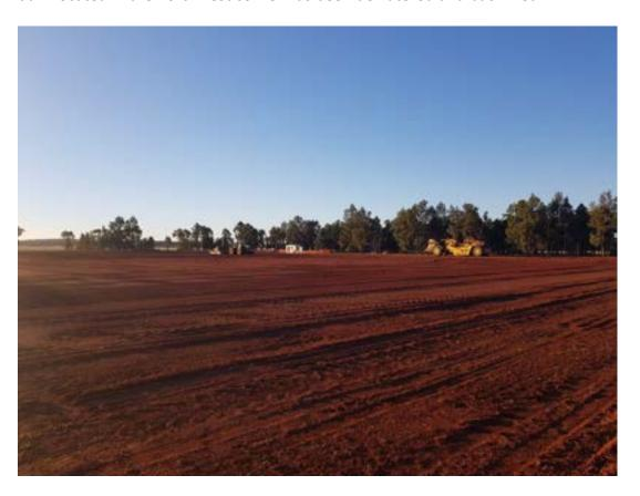
The decision to postpone construction until substantial rainfall had occurred has proven beneficial with soil conditions currently at or very close to optimum moisture content.
