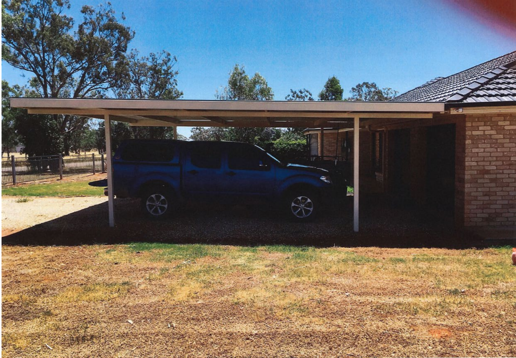
Photo 3: Side of Carport
