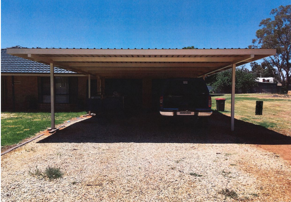
Photo 1: Front of Carport
